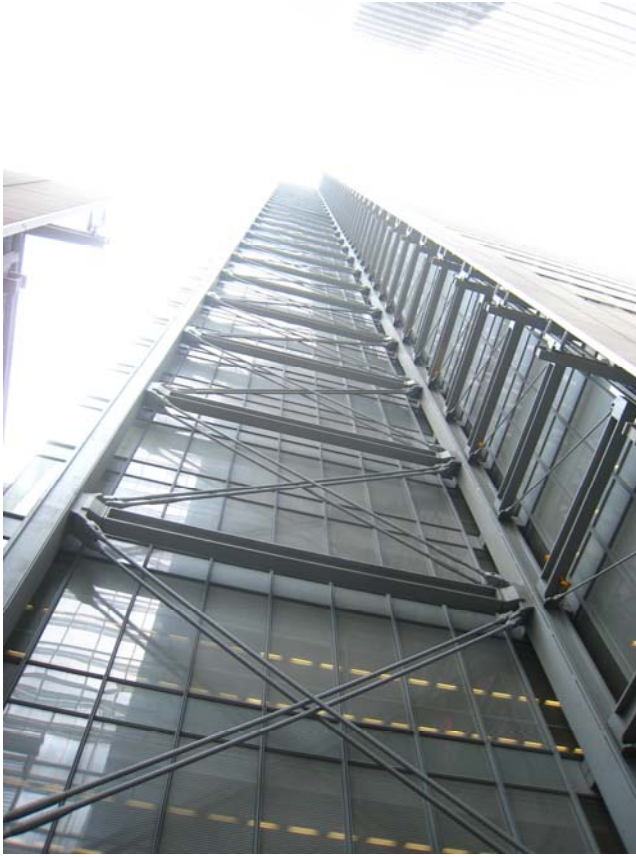
Figure 29: Exterior X-bracing
