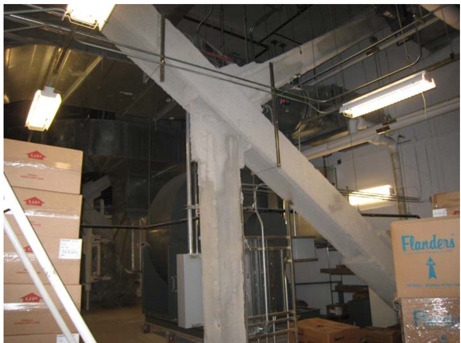
Figure 32: Outrigger on 28 th Floor
